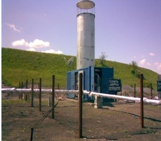
Figure 16 – The gas-utilizing compressor plant of container type
